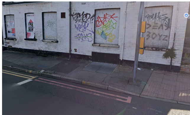
Figure 15 - Cellar door on Bedford Road frontage
